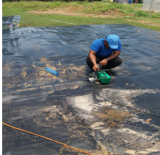
On Site Welding of HDPE pond liner
