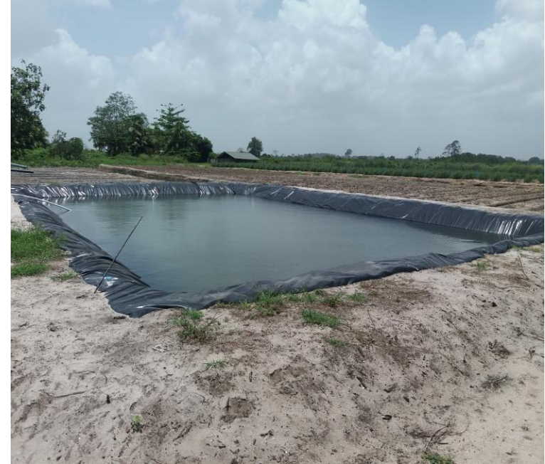
Water reservoir 20x12x2m lined with pond liner
